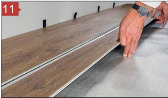
STEP 11: Disassembling the long side As you go, don't forget to use a rubber mallet on the short sides to secure the locking.
